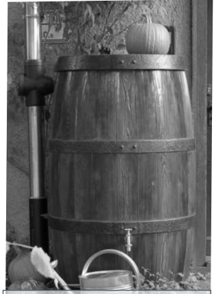
\* **Top Tip!** Before filling with water, check the drain-down points are fully tightened. They may just need a ¼ turn. A 2p piece is the perfect tool if you don't have the right sized screwdriver.
